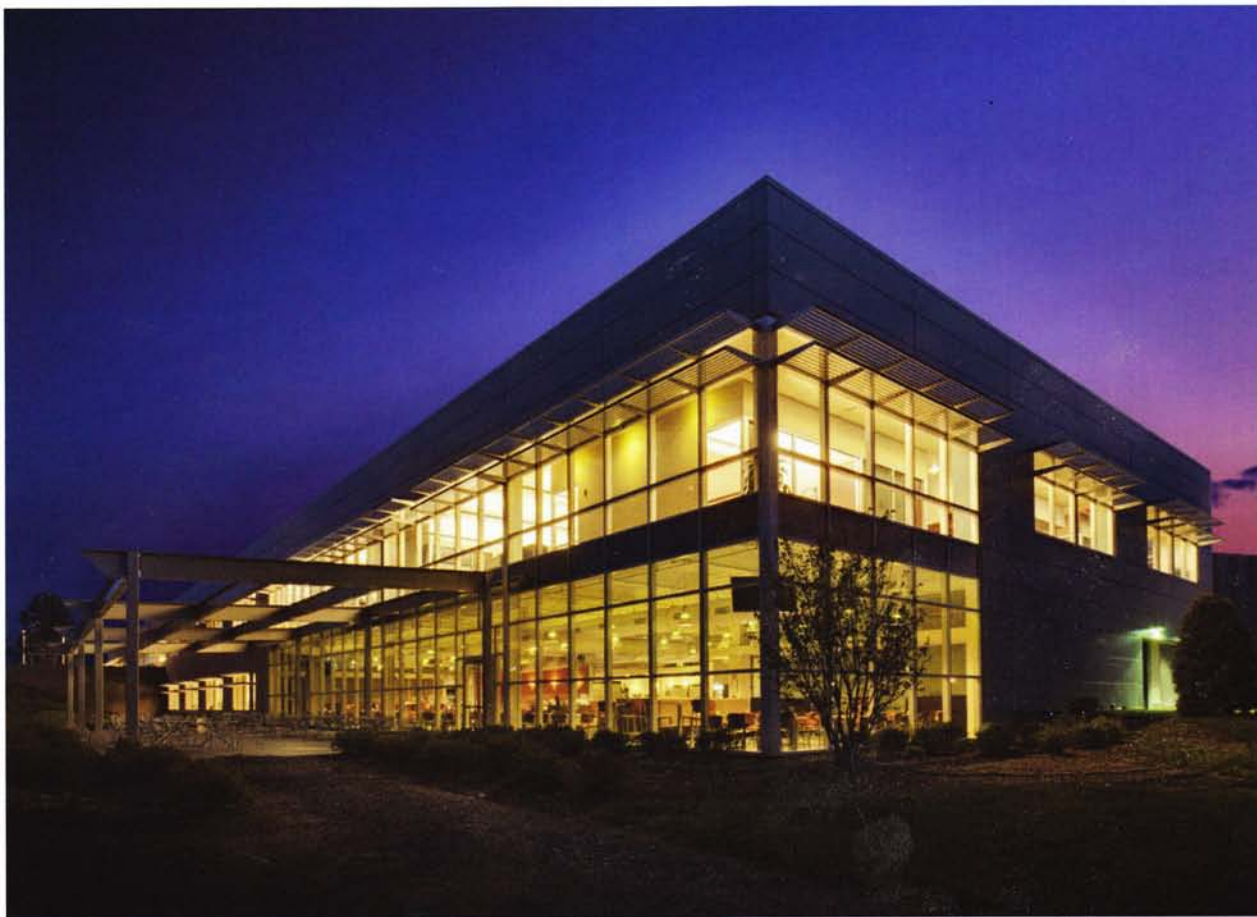
Welch-Allyn's newly expanded headquarters in Skaneateles Falls boasts a fitness area, full-service staff cafeteria, and is expected to receive LEED gold certification. Photo courtesy of Welch-Allyn.
